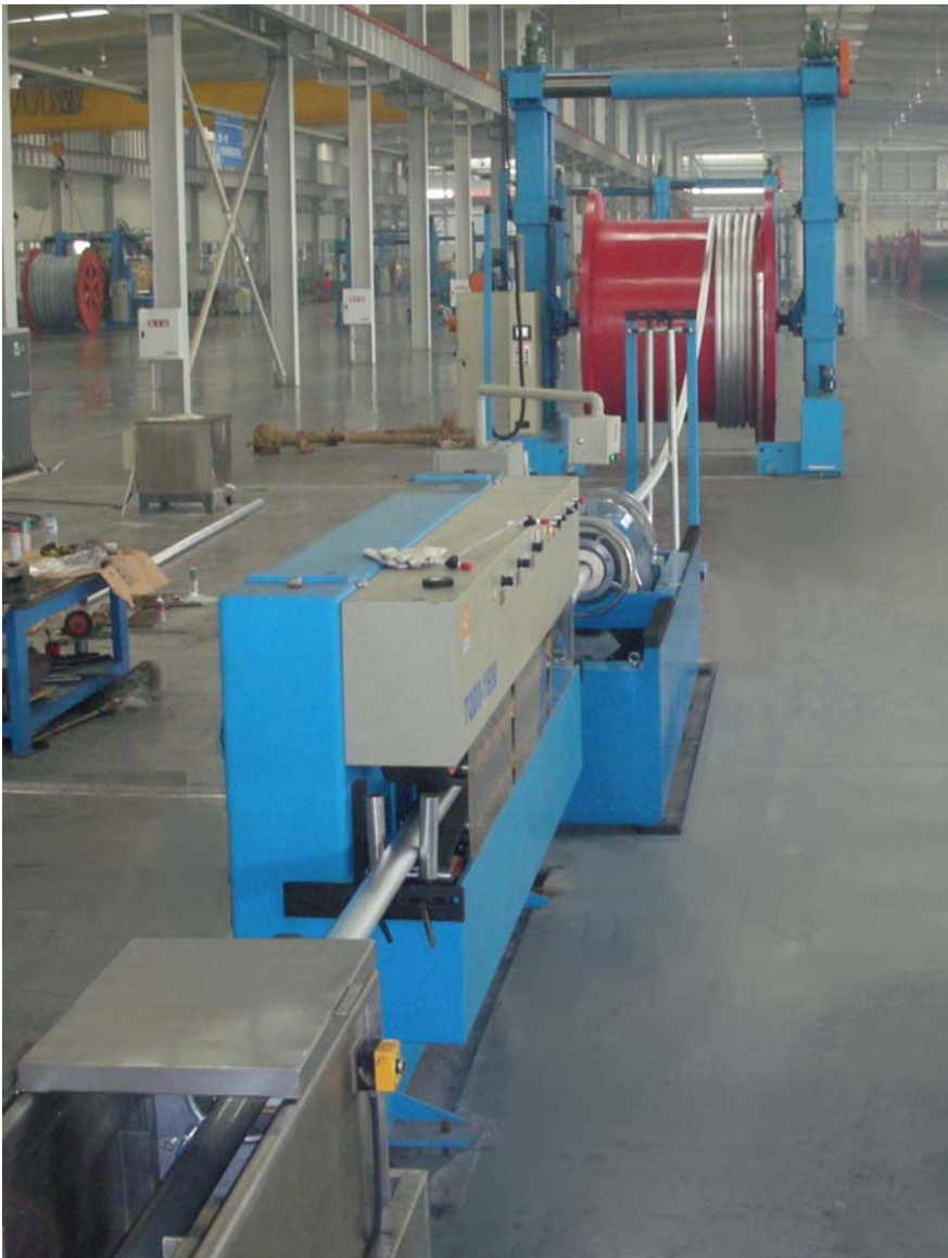
Sheathing of 86mm Cable
